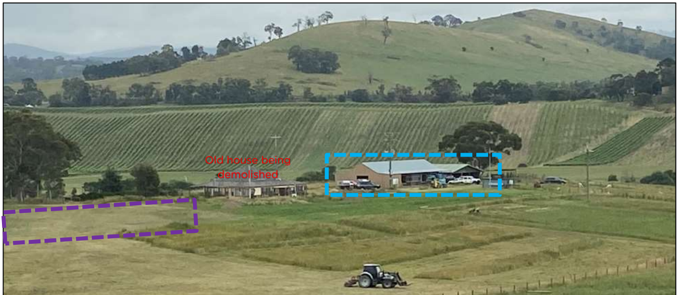
Figure 3.3 Existing Buildings to be used for distillery, café and functions
