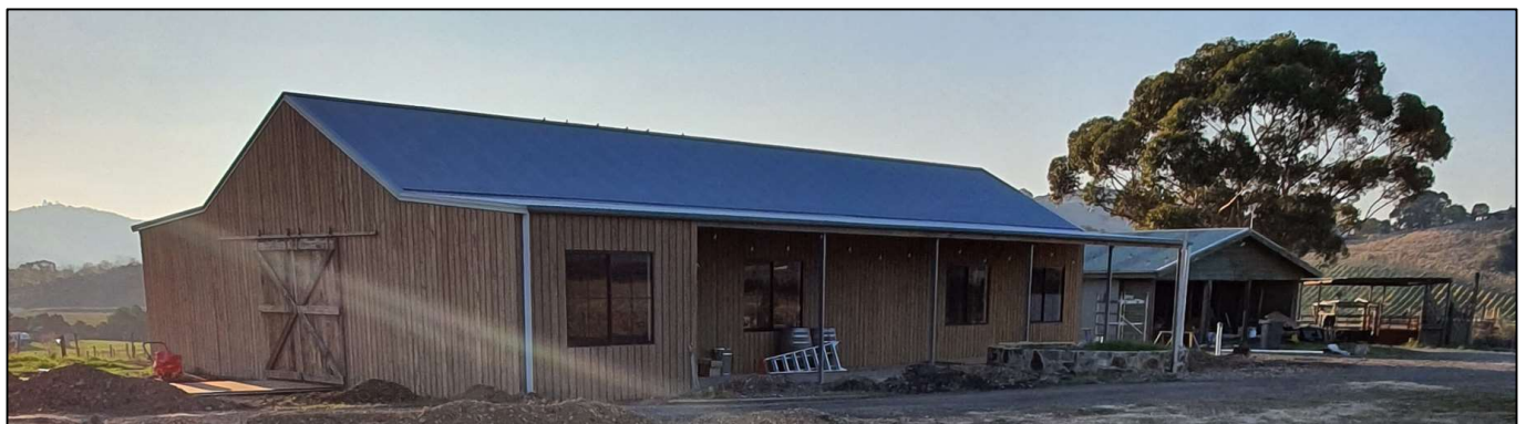
Figure 3.4 Existing Buildings (Shed 1 left / Shed 2 right) Source: client photo (April 2022)
